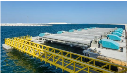
Synchro Lift is designed to accommodate vessels of 70.0 meters LOA in length with a weight of 2,200 tonnes.
