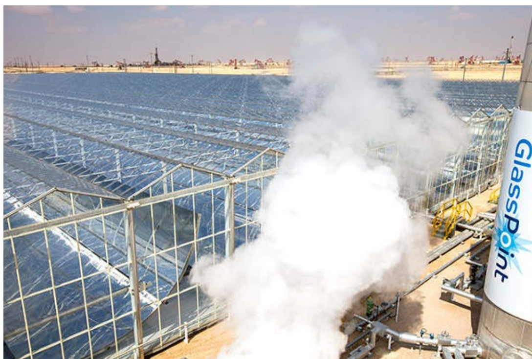
Miraah facility generates 6,000t/day of steam for use at Amal Oil Field
