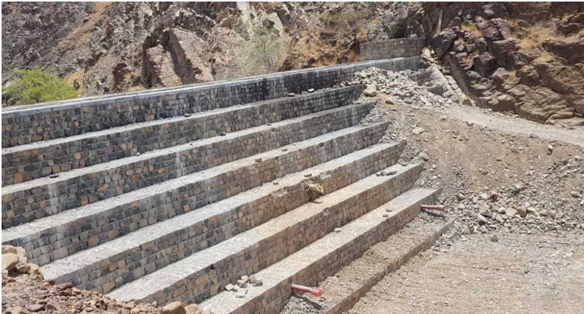
Underground recharge dam in Wilayat of Al Khaboura of Oman
