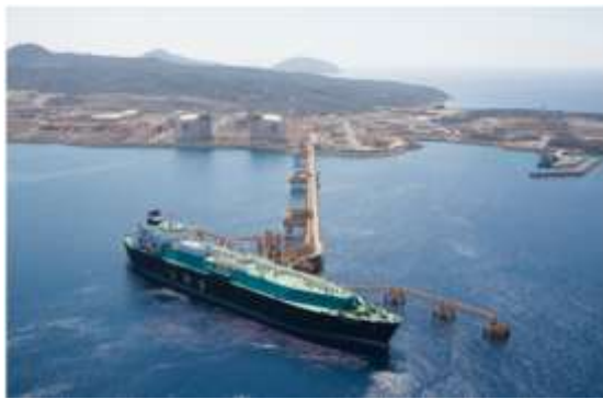
Balhaf (بلحاف) LNG Terminal in Shabwah (شبه) (Yemen LNG Co., Operations are suspended due to force majeure)
