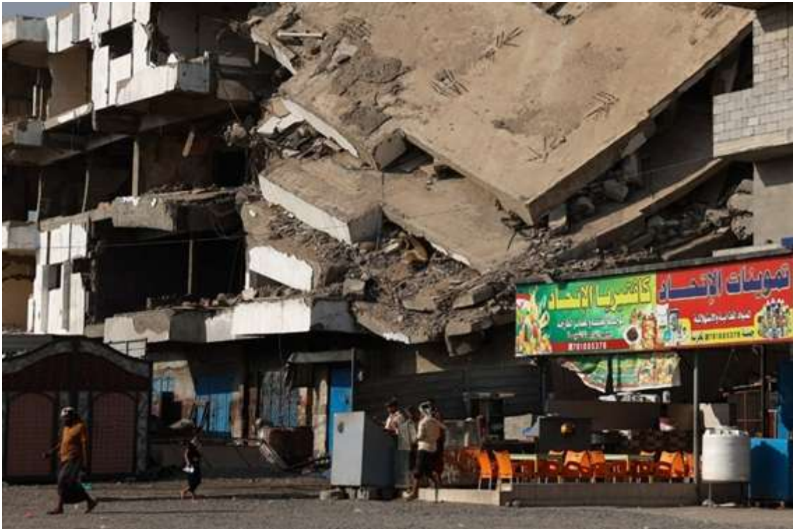
A restaurant located below a damaged building in Lahj province (October 15, 2025, Reuters)
